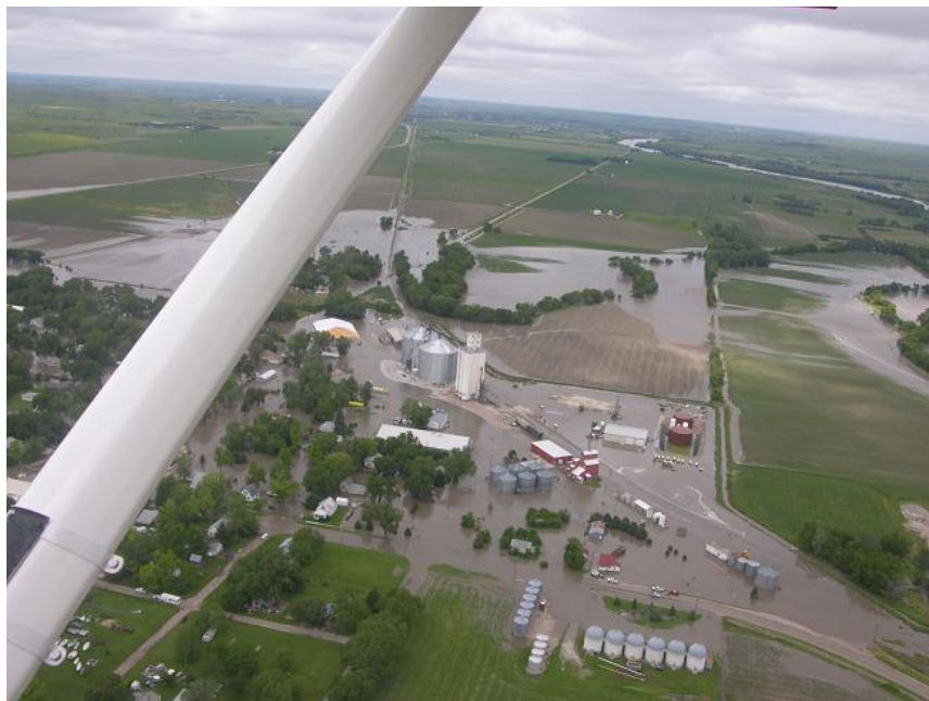
Aerial photo of North Loup after dam failure
