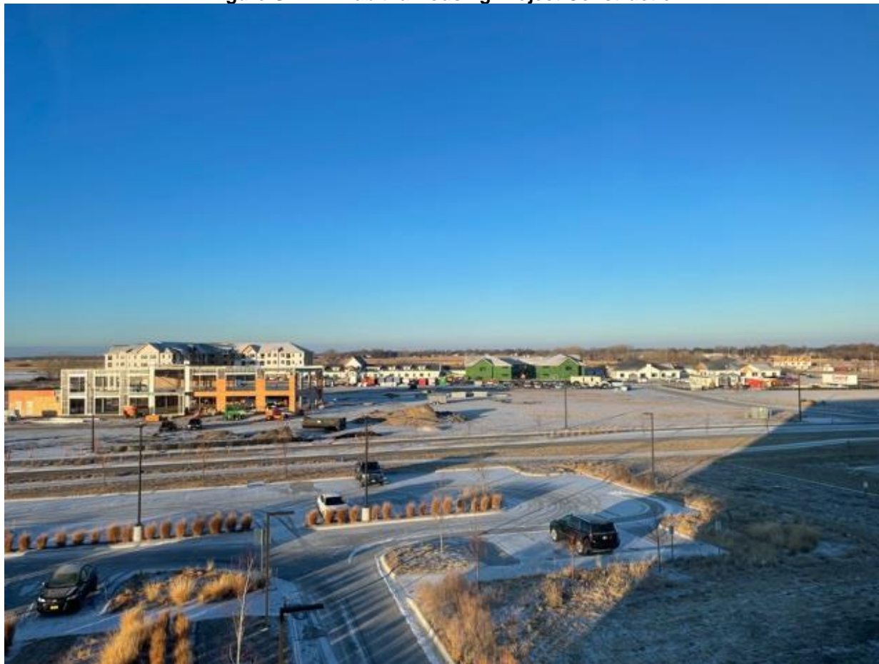
Figure GRA.4: Tabitha Housing Project Construction
