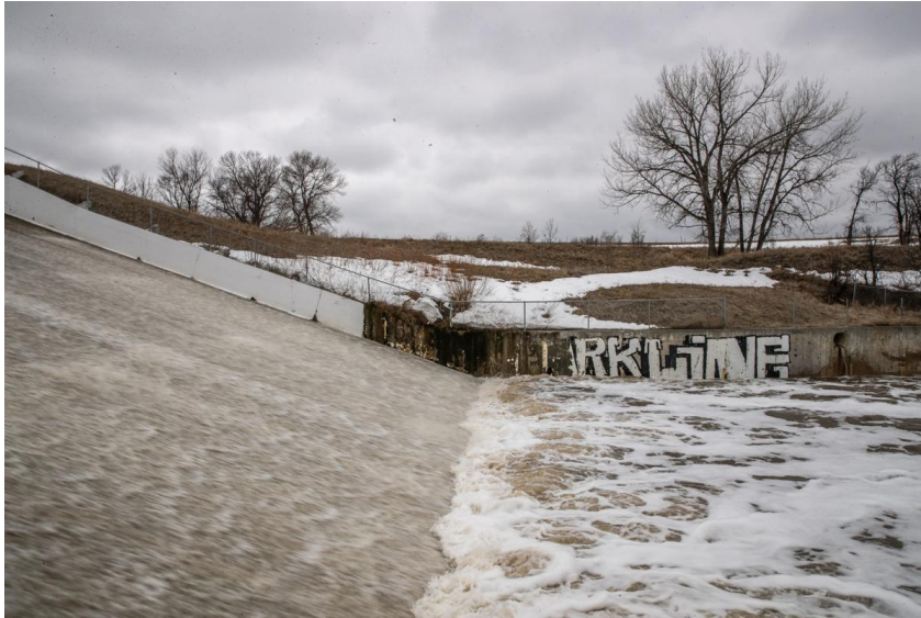
FIGURE 24: WATER FLOWS OVER WHITE CLAY DAM SPILLWAY
