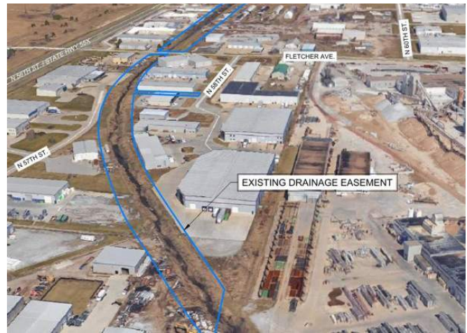
Easement encroachment along the channel
