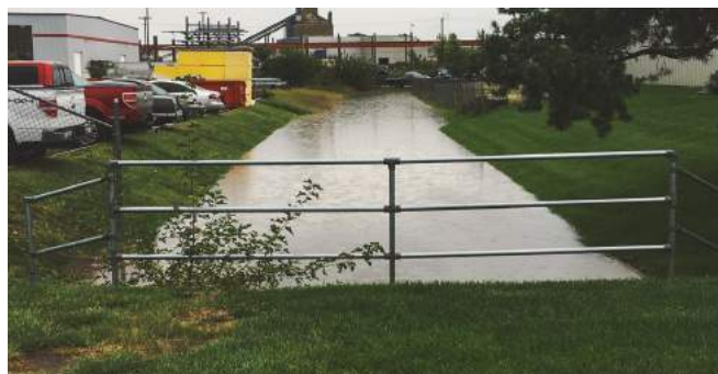
High water levels in the channel
