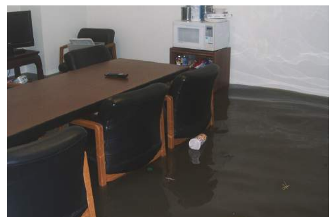
Flooded offices in the 56th and Morton complex
