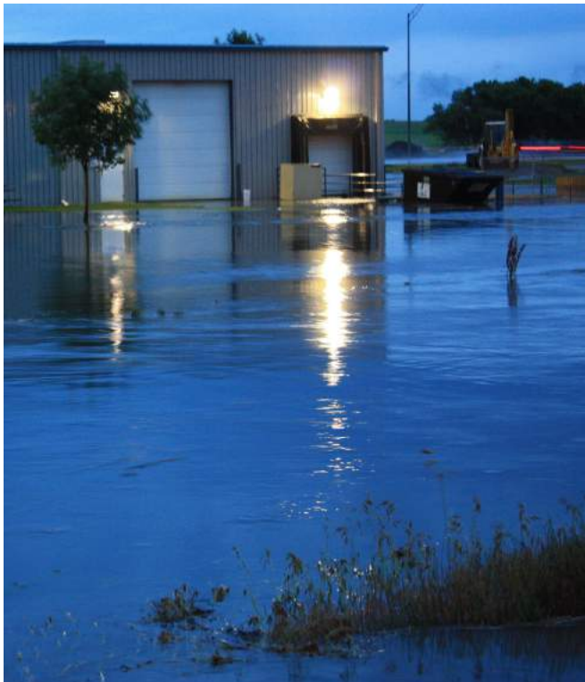
Water levels rise in the 56th and Morton complex
