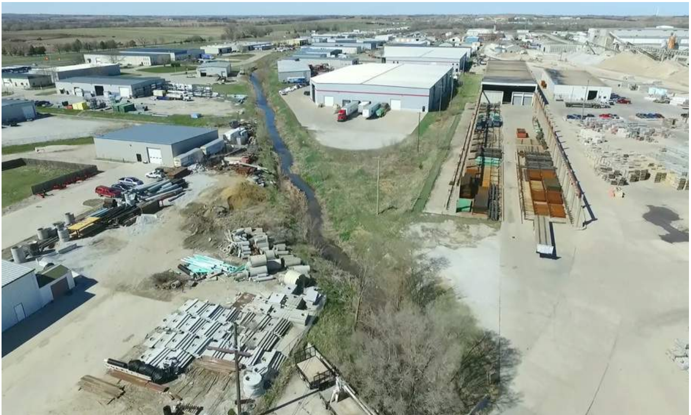
Aerial view of the drainage channel
