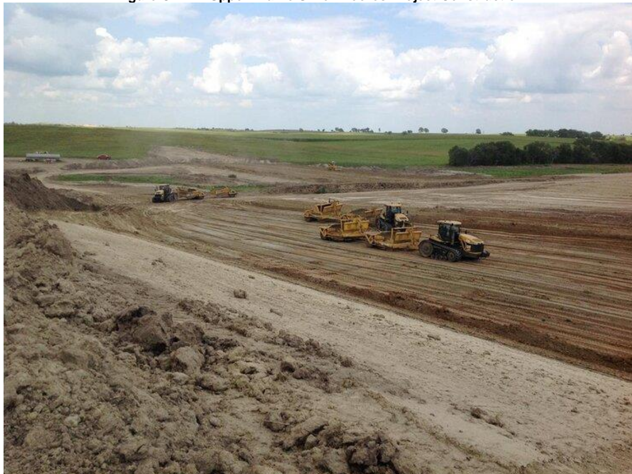
Figure CPN.4: Upper Prairie Silver Moores Project Construction
