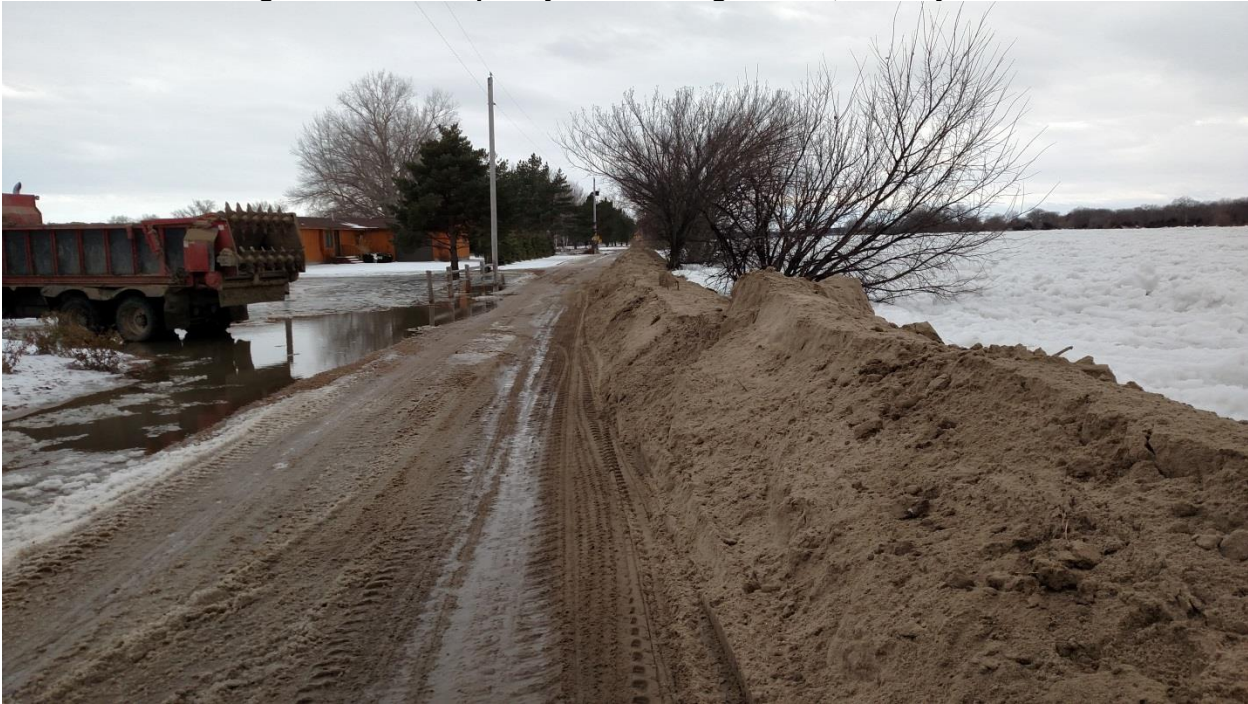
Figure MER.6: Temporary Berm During Ice Jam, January 2016
