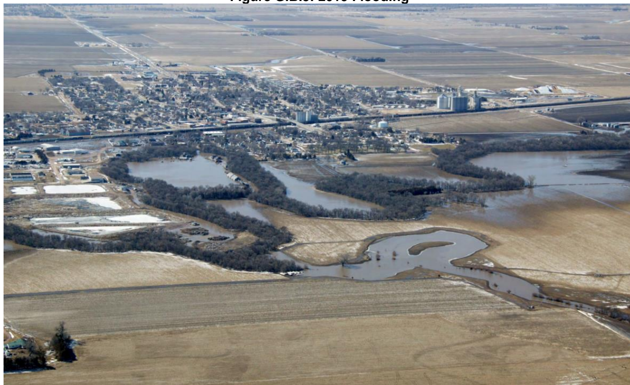
Figure GIB.5: 2019 Flooding
